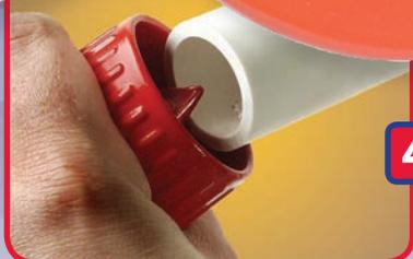
4 Use inside/outside Deburring Tool (Uniweld #70079) to remove burrs from pipe.
