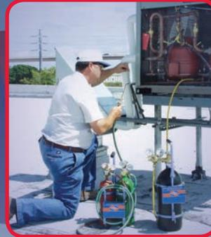
Purge and pressure test an A/C&R system
